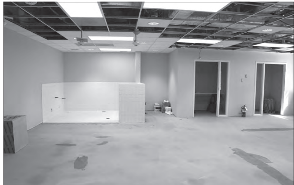
The new pre-school classroom floorplan will eliminate blind spots by moving the bathrooms and closets along the wall. In June, crews began the tile work in the bathroom area. The classroom is expected to be complete in mid-July.
