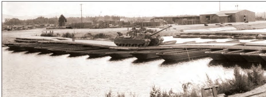
ABOVE: The U.S. Army Corps of Engineers opened the Yuma Test Branch near the present site of the proving ground below Laguna Dam on the Colorado River in 1943. This location was considered an ideal spot for testing portable combat bridges because of the abundance of swift flowing water that engineers could control. BELOW: Camp Laguna was one of 12 major U.S. Army desert training camps in the California-Arizona Maneuver Area, an 18,000 square mile area chosen by then-Maj. Gen. George S. Patton. Upwards of 15,000 troops were stationed at Camp Laguna at any one time for periods generally lasting six months. (U.S. Army photos)
