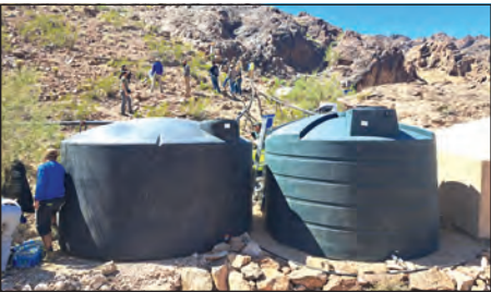
LEFT: “The new system we put in at this site is 23,000 gallons, and we put the catchment in an area with a pretty good catch basin that should be able to fill it with a decent rain event. When it gets completely full, it should be able to stay full for a couple of years,” said Daniel Steward. RIGHT: Wildlife officials are meticulous about keeping the drinkers a viable and perennial presence on the range. This past winter, YPG personnel joined up with the Arizona Department of Game and Fish and dozens of volunteers to upgrade the massive tanks that store water for drinkers at two locations: one saw work done in January, the other in March.
