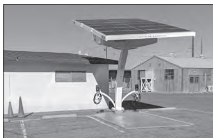
U.S. Army Garrison Yuma Proving Ground installed three solar-powered chargers for electric vehicles on post. These chargers are to be utilized by government vehicles only, per the Army's Installation Management Command guidance. (Photo by Reinhard Brenneis)
