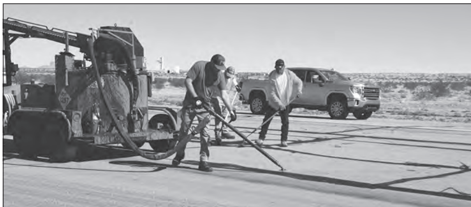
Laguna Airfield is undergoing improvements. All the pavements are being resurfaced in one way depending on their needs. Cracks are being filled and fog sealed on the runways, taxiways, and aprons. (Photos by Ana Henderson)
