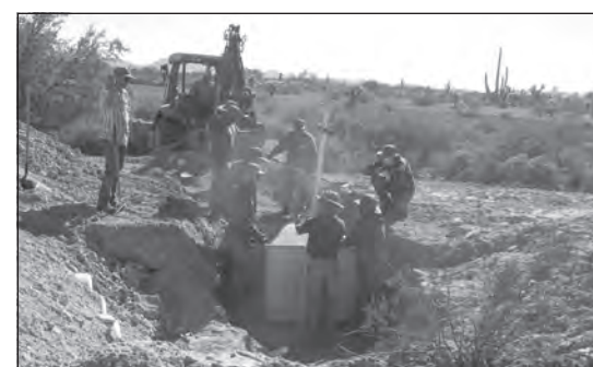
The Arizona Game and Fish Department with the help of Yuma Proving Ground (YPG) and volunteers constructed a new wildlife water catchment on YPG's East Arm in late January. The Xamool Tank was designed, and placed to benefit Sonoran Pronghorn and can hold up to 22,000 gallons of rain water. (Photos by John Kulberg)
