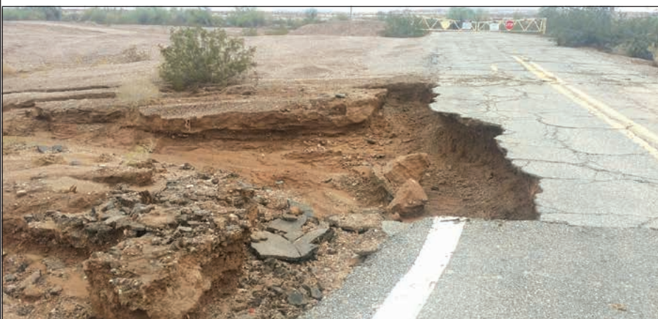
Monsoon season in the Desert Southwest usually means thunderstorms, strong winds, torrential rain and haboobs. This road damage caused by monsoon rain in 2018 is typical of the damage torrentials rain cause at YPG.
