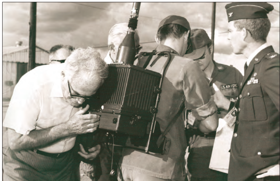
GPS testing started with bulky equipment in the 1970's by the early 1980s, GPS technology had been miniaturized to the point that a man portable backpack weighing a mere 25 pounds began testing with Soldiers at the proving ground. (U.S. Army photo)
