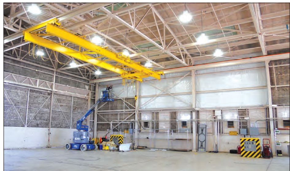
The original exposed insulation is being removed and replaced with modern vapor barrier insulation that will resist moisture and pests. (Loaned photo)
