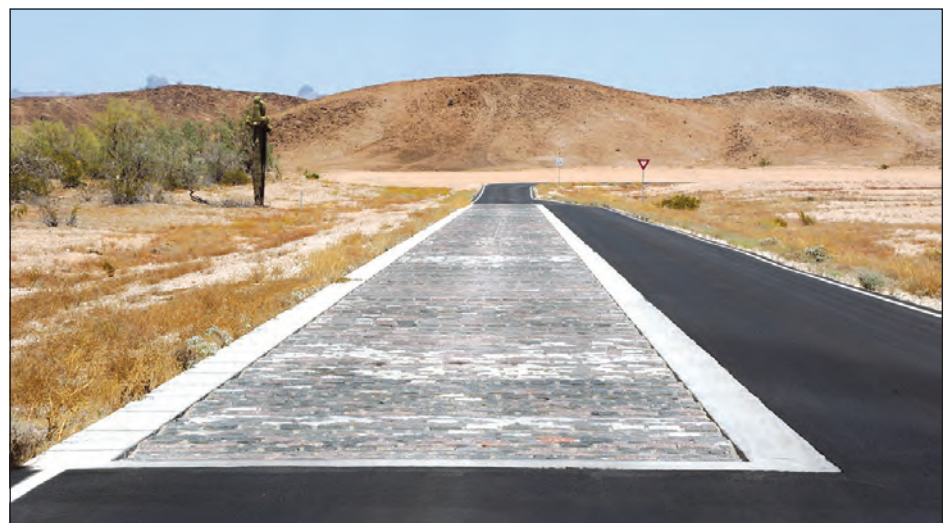
GM's test track includes a variety of punishing road conditions, and the Belgian block course is particularly jarring to passengers in a vehicle. (Photos by Mark Schauer)
