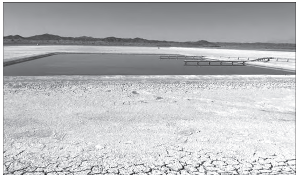
Over the years of waste accumulation, a lagoon needs to undergo a deep cleaning. The main lagoon currently has been pumped and drained. The drying phase will produce a strong sewage smell but will be alleviated as the drying progresses.
