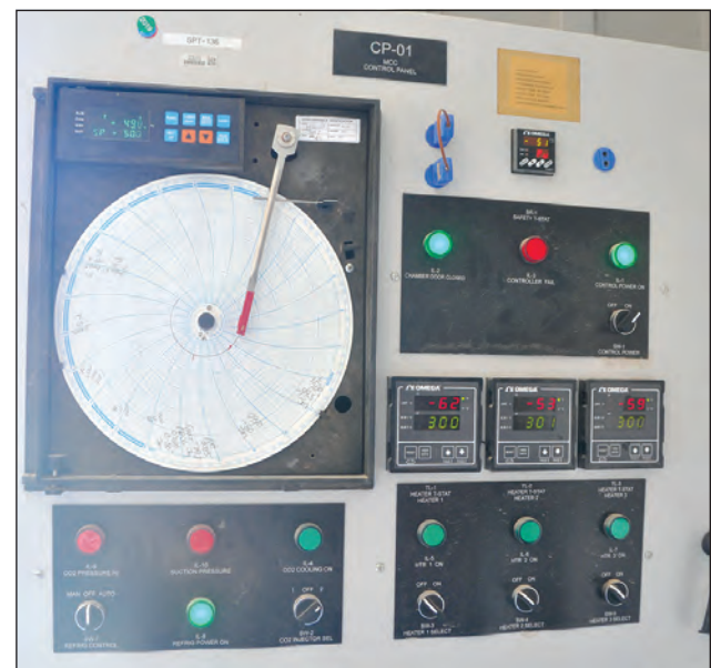
In addition to transporting ammunition, conditioning chamber personnel constantly monitor the chamber's carbon dioxide (CO2) levels used to maintain the cold temperatures.
