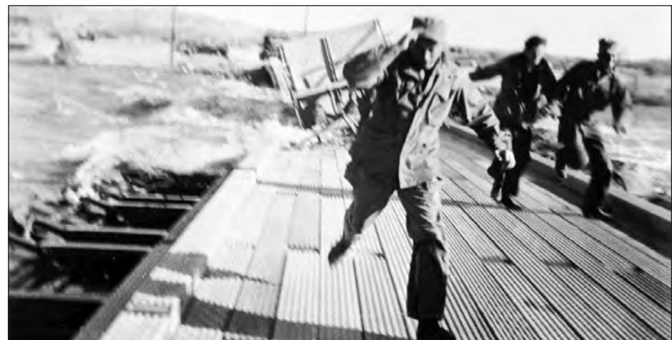
Even under controlled conditions, bridge testing at Yuma Test Station was dangerous work, as seen here. "We had two M4 tanks that registered about 32 tons each," Banning recalled. "After we made sure it could hold the trucks up, we had a brave guy that would take a tank and creep out. His orders were, 'If you feel any slipping, put it in reverse and back off.'" (US Army photo)
