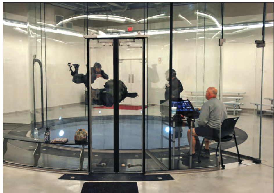
YPG's vertical wind tunnel can accommodate eight jumpers simultaneously with a top speed of 175 miles per hour. The nearly 100 foot-tall structure contains over 4,000 tons of concrete and 80 tons of steel. The building was completed in about a year, six months ahead of schedule, and 95% percent of the labor to build the $10.3 million structure came from within Yuma. (Photo by Mark Schauer)
