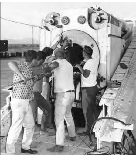
A gun crew loads the High Altitude Research Projectile gun at YPG prior to its record-setting projectile launch in 1966. The massive gun, constructed of two Navy 16 inch battleship tubes, fired 30 rounds between June and November of that year. (US Army photo)
