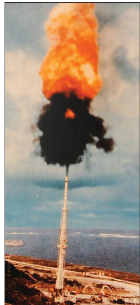
Of the three HARP guns that were built, only YPG's remains in usable condition. The gun built on the Caribbean island Barbados, seen here in 1966, has long since corroded. Private industry customers remain interested in the HARP for its original intended purpose of launching satellites into space. (Loaned photo)
