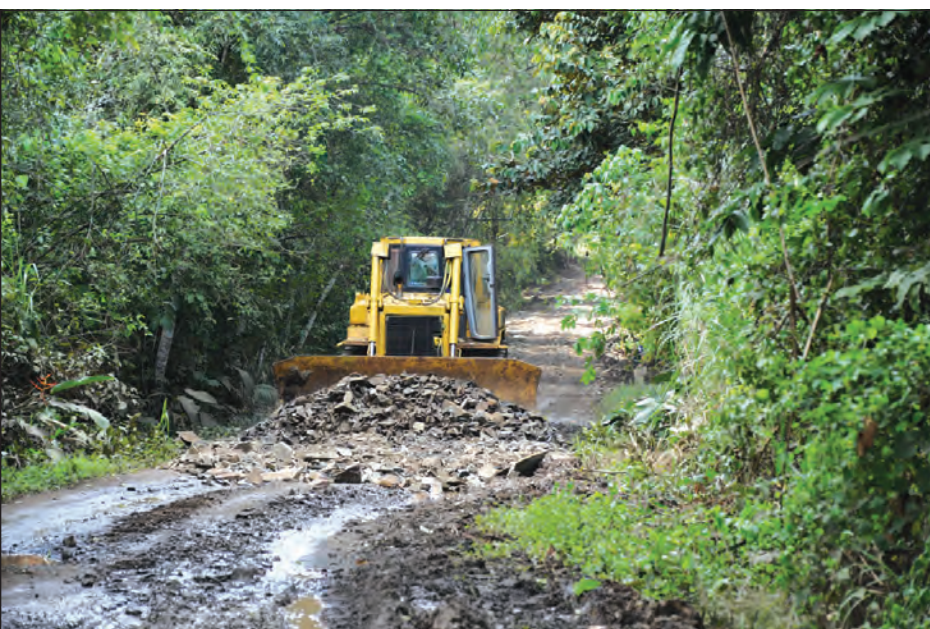
Extremely rugged in the best of circumstances, the profile of the facility's roads changed as the rains flooded and washed out trails more and more with each passing day. Roads had to be regularly reinforced with gravel material to keep them usable, as water-saturated soil will no longer compact. (Photo by Mark Schauer)
