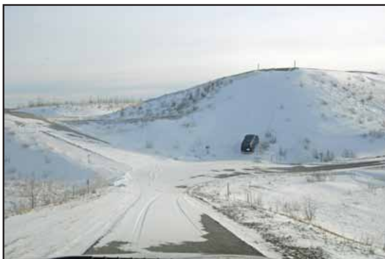
ABOVE: CRTC's Mobility Test Track boasts grades of up to 60%, as seen here. The steepest grade found on an interstate highway in the United States is 6%. (PHOTO BY MARK SCHAUER)
