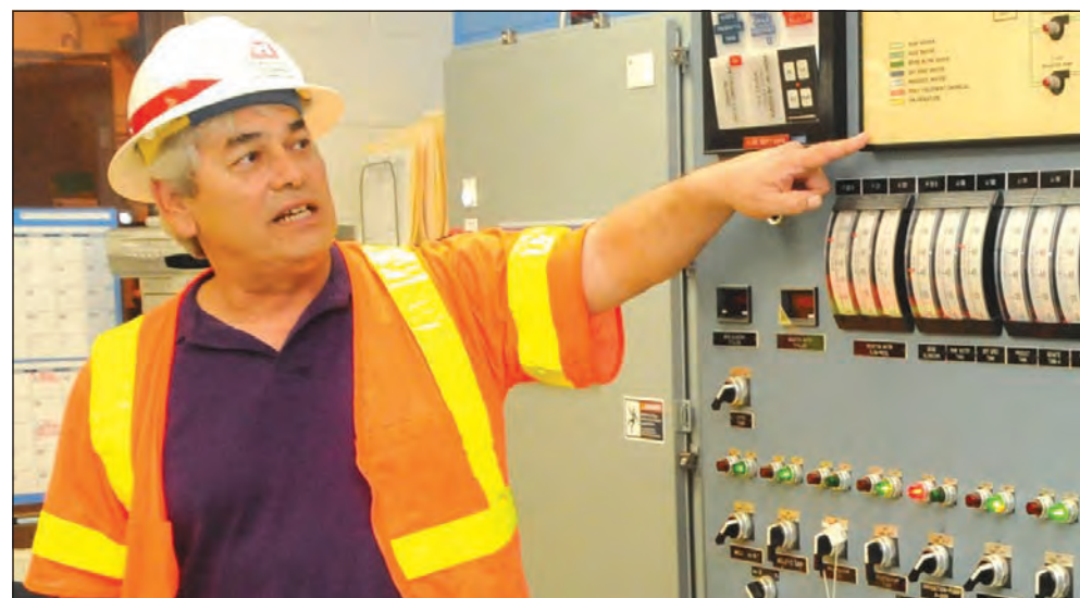
Ernesto Elias, Army Corps of Engineers project supervisor, shows the original control panel that took up an entire wall in the Howard Cantonment Area's water treatment plant. In service since 1987, replacement parts for the panel's gauges are no longer available on the commercial market, which necessitated a substantial overhaul of the facility's infrastructure. (Photo by Mark Schauer)
