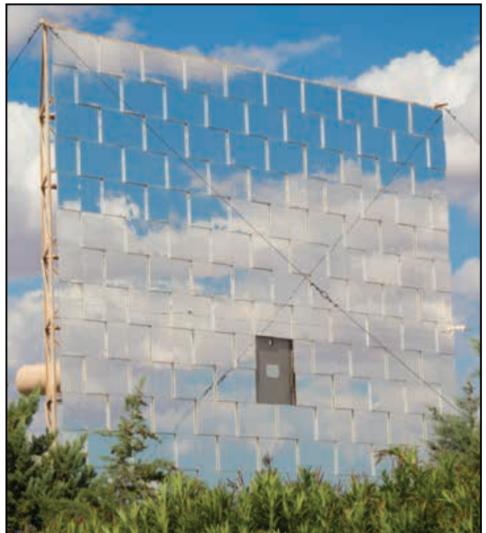
White Sands Solar Furnace (WSSF) uses mirrors to concentrate sunlight and achieve temperatures of 5000 degrees F. This intense heat can be pulsed to duplicate the thermal effect of a nuclear weapon detonation. (Photo by G. Palombit)
