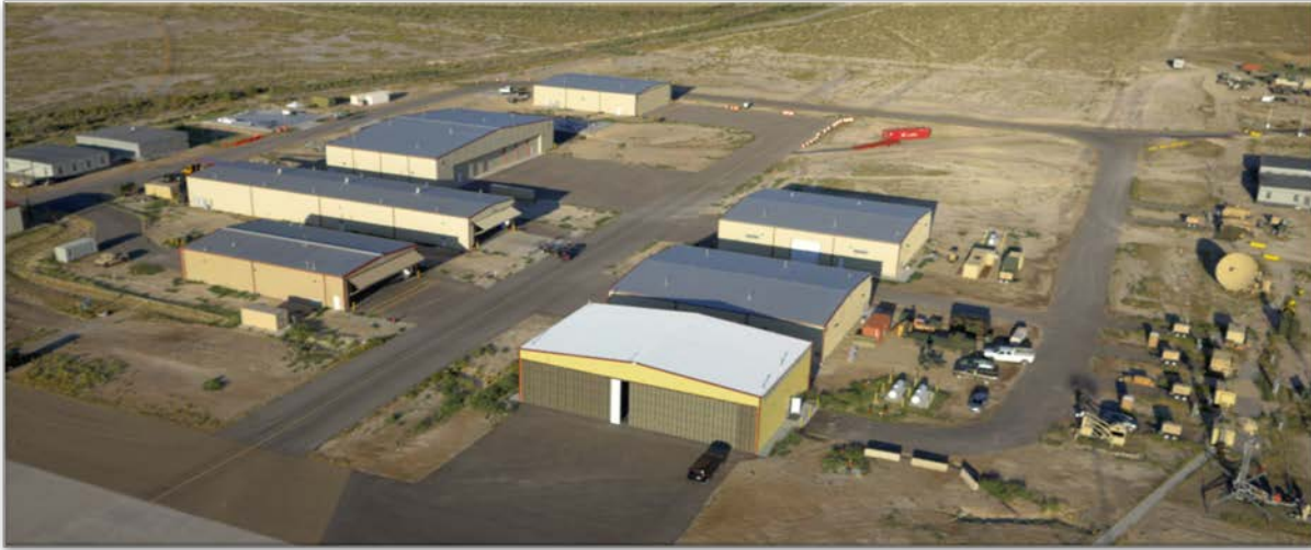
FIGURE 4: RIAC HANGER FACILITIES
