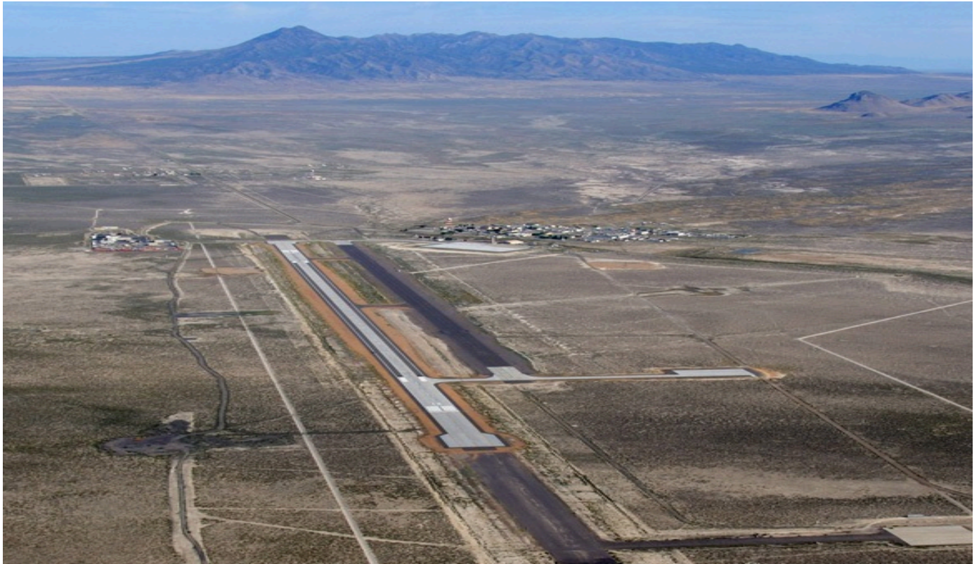
FIGURE 2: MICHAEL ARMY AIRFIELD
