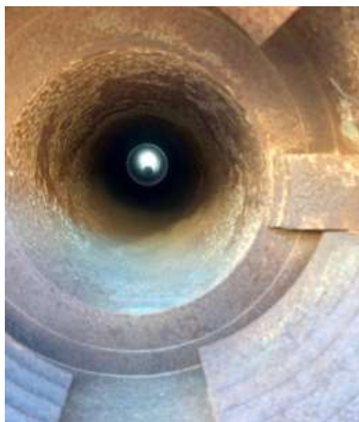
Looking from the breech to the muzzle of the 23 1/2-foot barrel of the naval gun in the desert of Dugway Proving Ground. The bore is 6 inches in diameter; it once fired projectiles weighing 95 to 98 pounds, depending upon use. Photos by Col. Scott Gould
