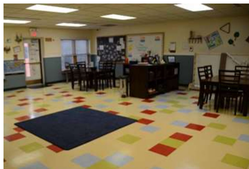
The renovated areas of the Child and Youth Services building are bright and cheerful, offering Dugway children a welcoming place to go for childcare, school liaison services, instructional programming and before- and after-school activities.
