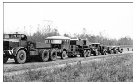
A 25-ton 6 x 6 truck tractor undergoes a field dynamometer test, November 1947.
