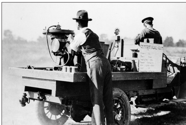
Testing a smooth bore centrifugal gun at Aberdeen Proving Ground, circa 1918. The gun proved to be highly inaccurate.
