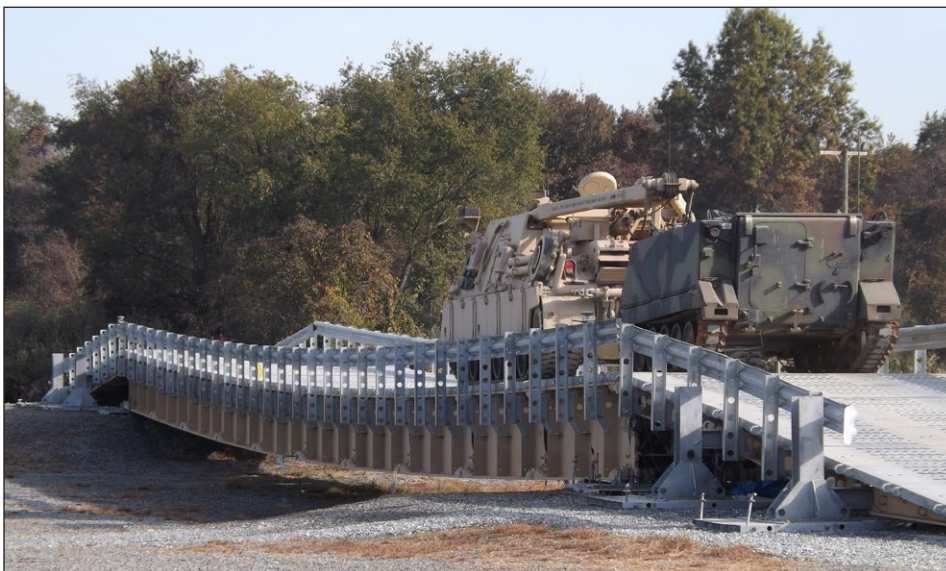
Bring it on! The M88 armored recovery vehicle tows an M113 personnel carrier across the LOCB. Military load classification for the LOCB is 120 wheeled/100 tracked in normal cross; 150 wheeled/120 tracked in caution cross.
